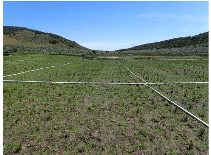
One of the completed wetland restoration areas
