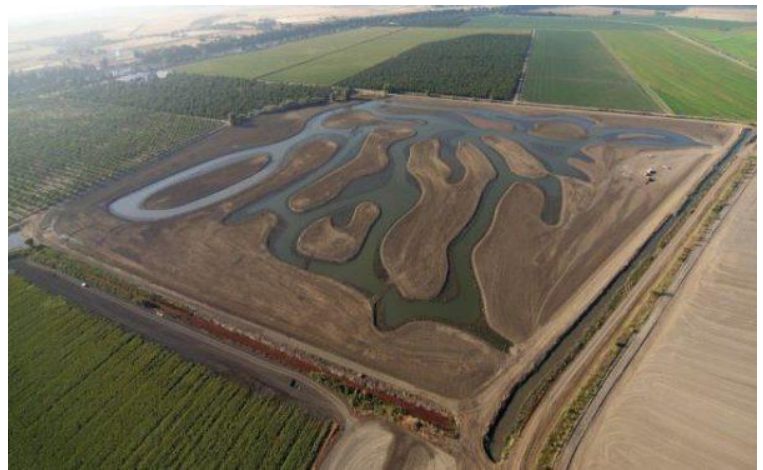
River Ranch Wetlands After Construction 2013
